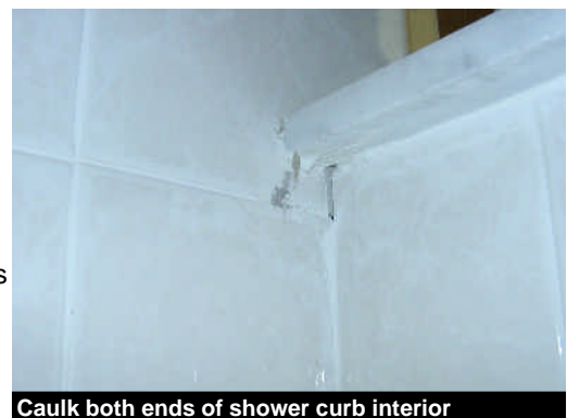
Caulk both ends of shower curb interior
